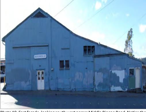
Photo 19. East façade, looking south west across Middle Rincon Road. Notice the air vents and large rolling barn doors. These are typical features of a feed mill.
