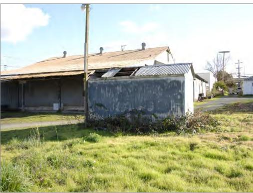
Photo 28. North façade of shed, looking south. Notice the missing metal sheets on the roof.
