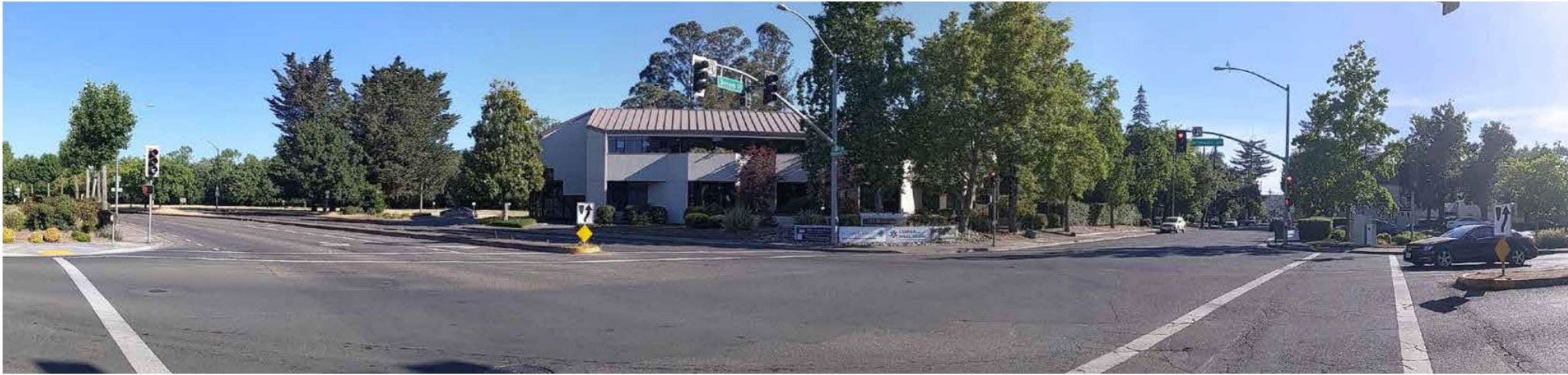
1 CORNER OF 2ND STREET AND BROOKWOOD AVENUE LOOKING SOUTH
