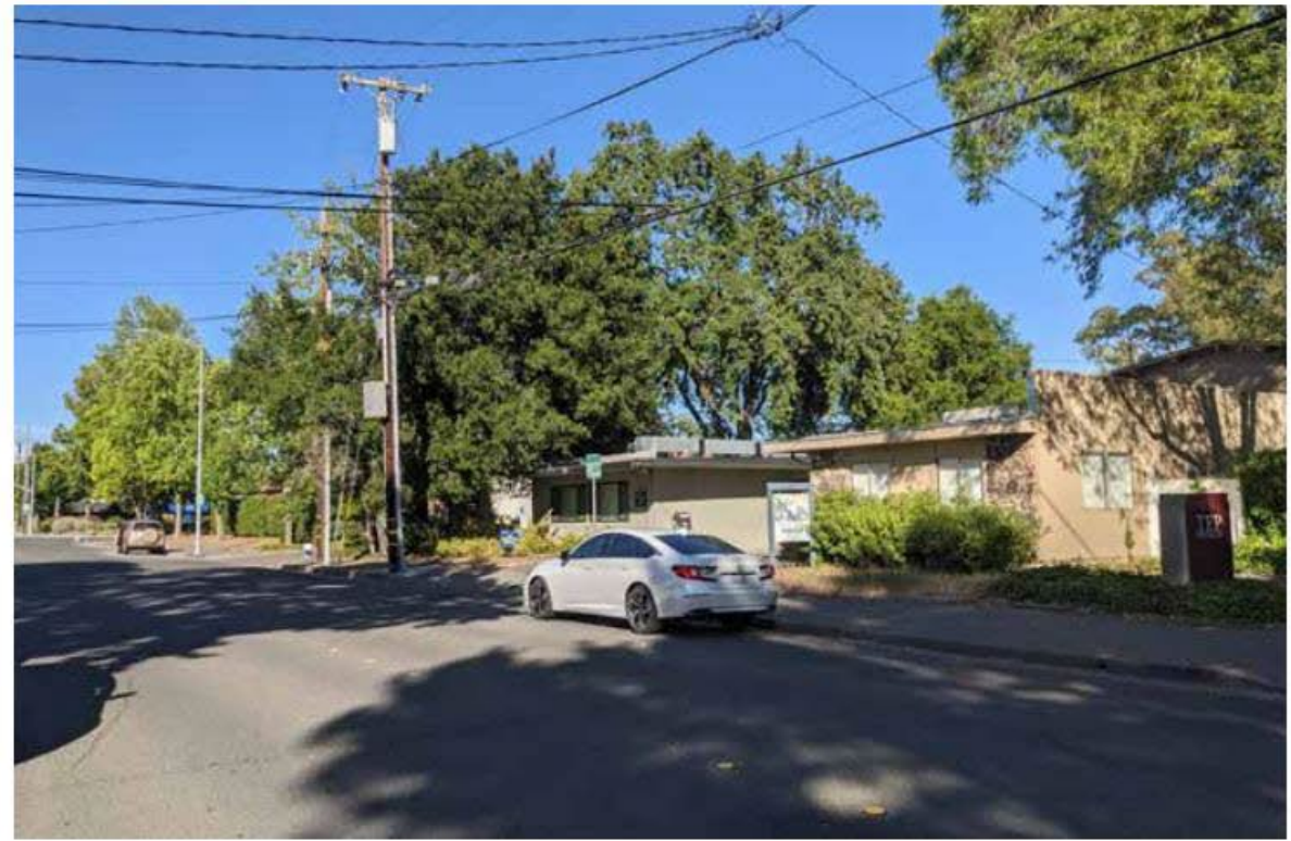
6 2ND STREET LOOKING NORTHEAST
