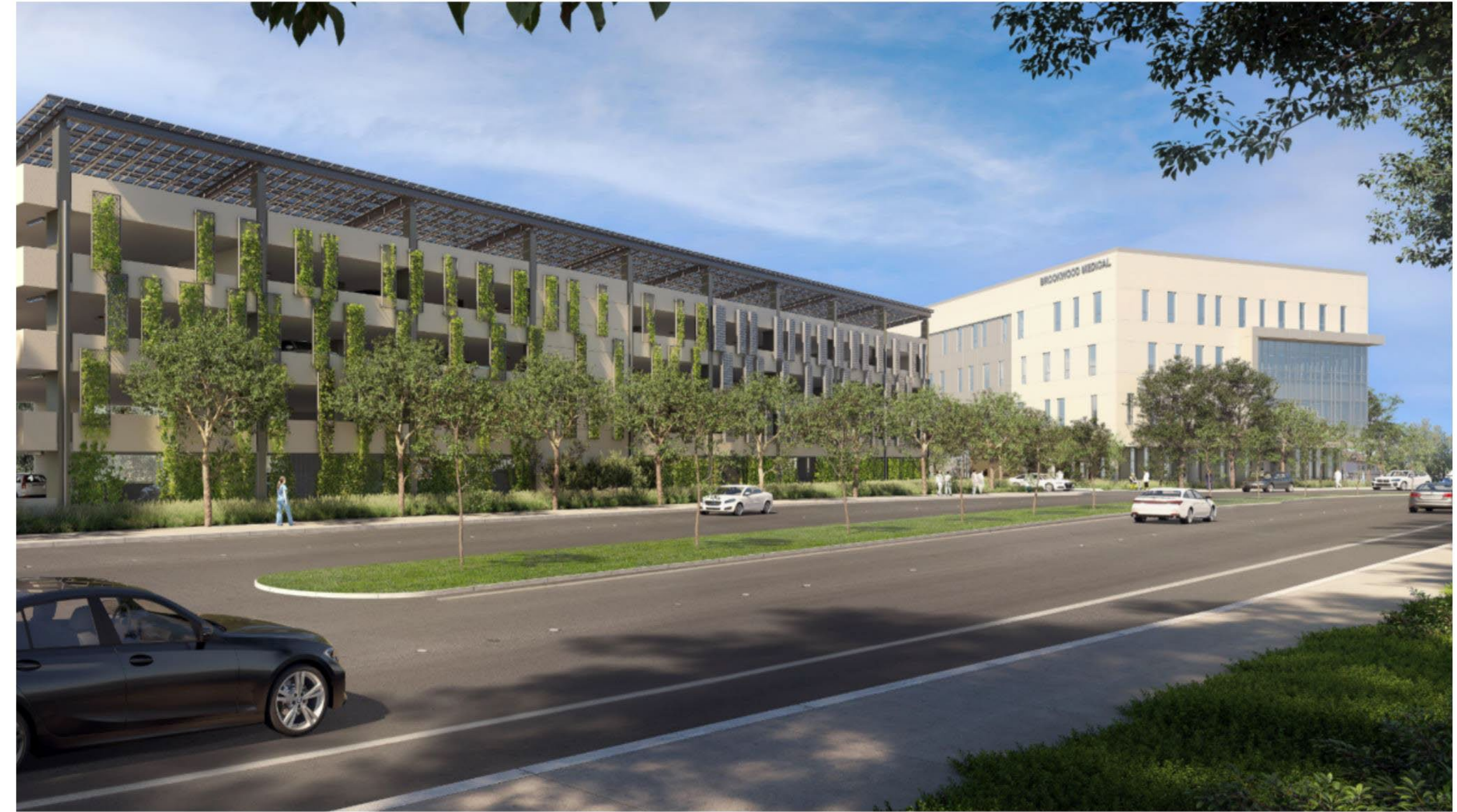
BUILDING CORNER - EAST 1
