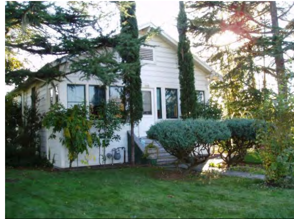
FIGURE 4. HOUSE AT 1200 HEARN AVENUE.
