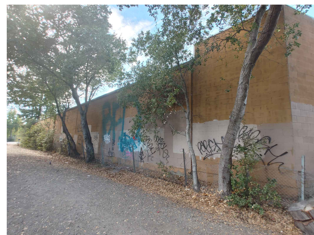
10 A-1 SOUTH WALL OF APN 015-390-049 (NOT IN PROJECT SCOPE)
