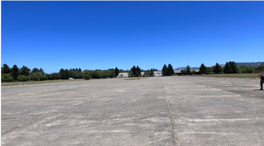
Photograph 3: Facing east across full site.
