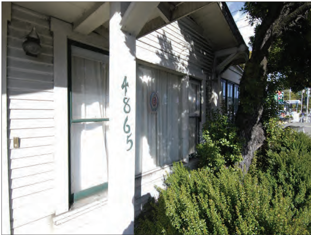
Photo 6. Double hung wood windows on the primary south façade, looking northeast.
