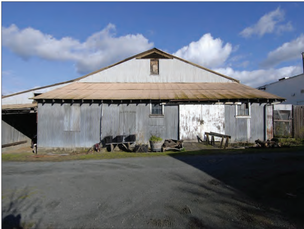
Photo 25. Lean-to on the west façade with two wood framed windows and a sliding barn door, looking east.
