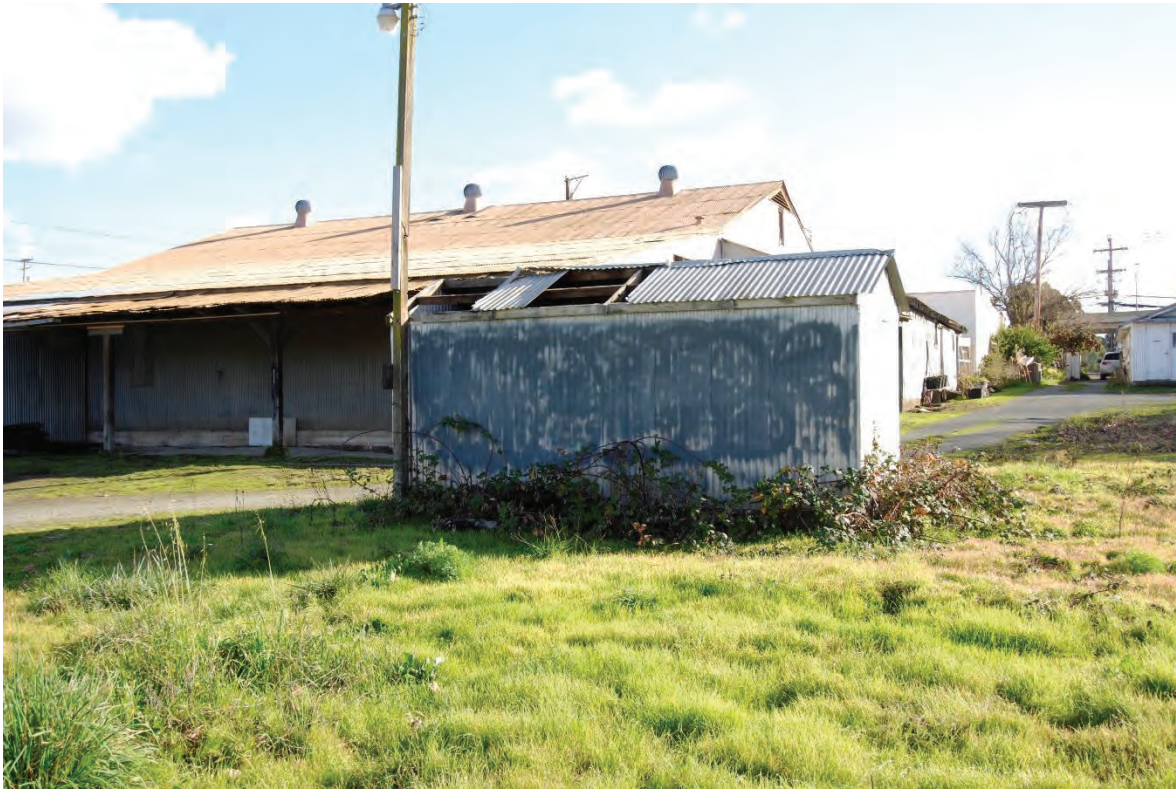
P5b. Description of Photo: North façade of utility shed, looking south. Notice the missing metal sheets on the roof.
