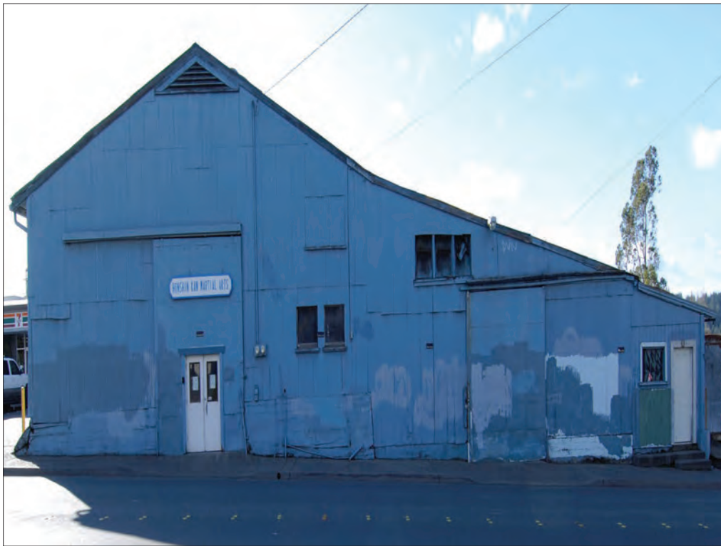
Photo 19. East façade, looking south west across Middle Rincon Road. Notice the air vents and large rolling barn doors. These are typical features of a feed mill.
