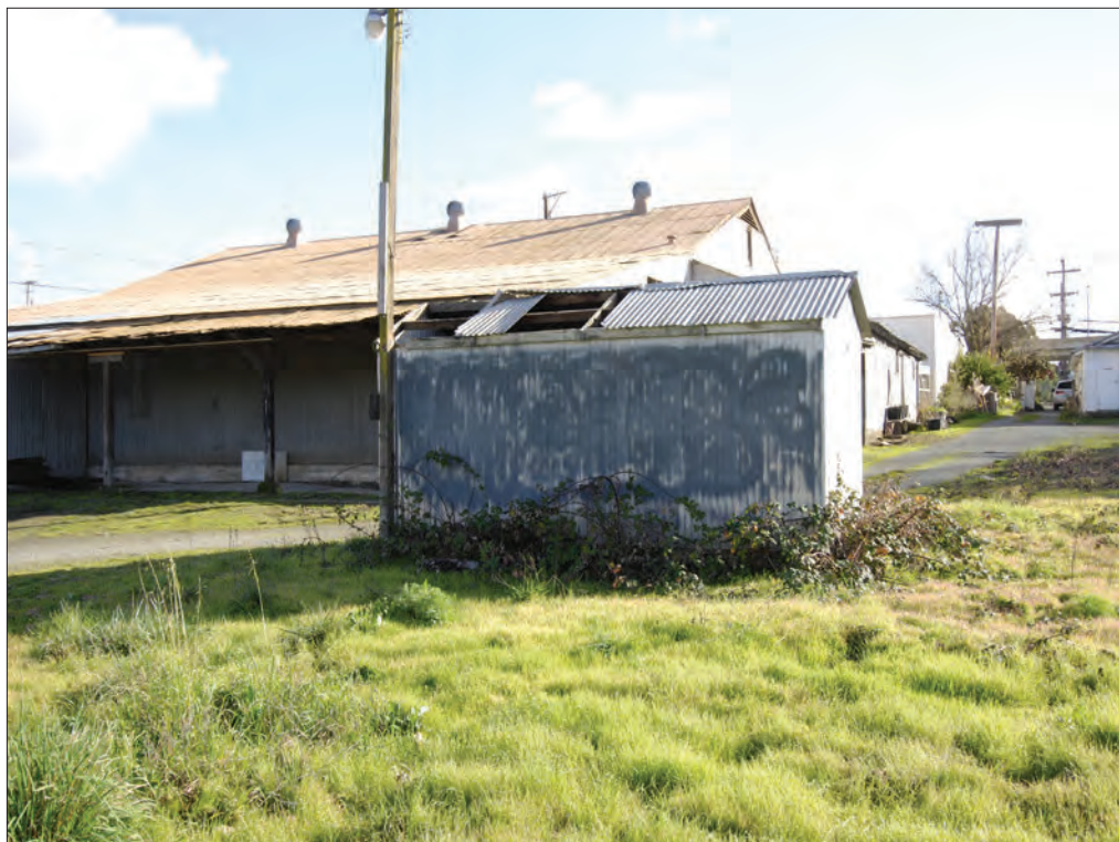
Photo 28. North façade of shed, looking south. Notice the missing metal sheets on the roof.
