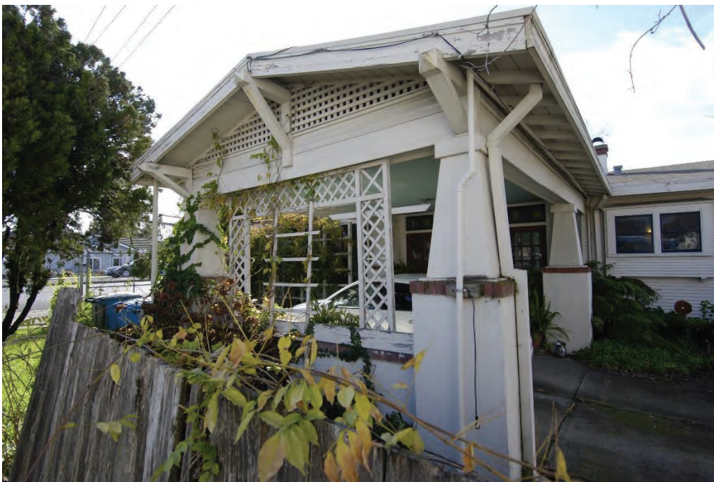
P5b. Description of Photo: Porte cochere on the east façade with tapered piers atop concrete pedestals with brick details, looking west. Note the triangular knee braces in the wide eave overhang.
