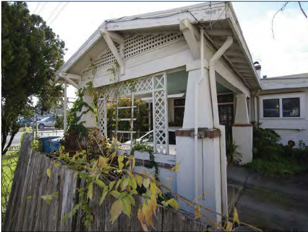
Photo 7. Porte cochere on the east façade with tapered piers atop concrete pedestals with brick details, looking west. Note the triangular knee braces in the wide eave overhang.
