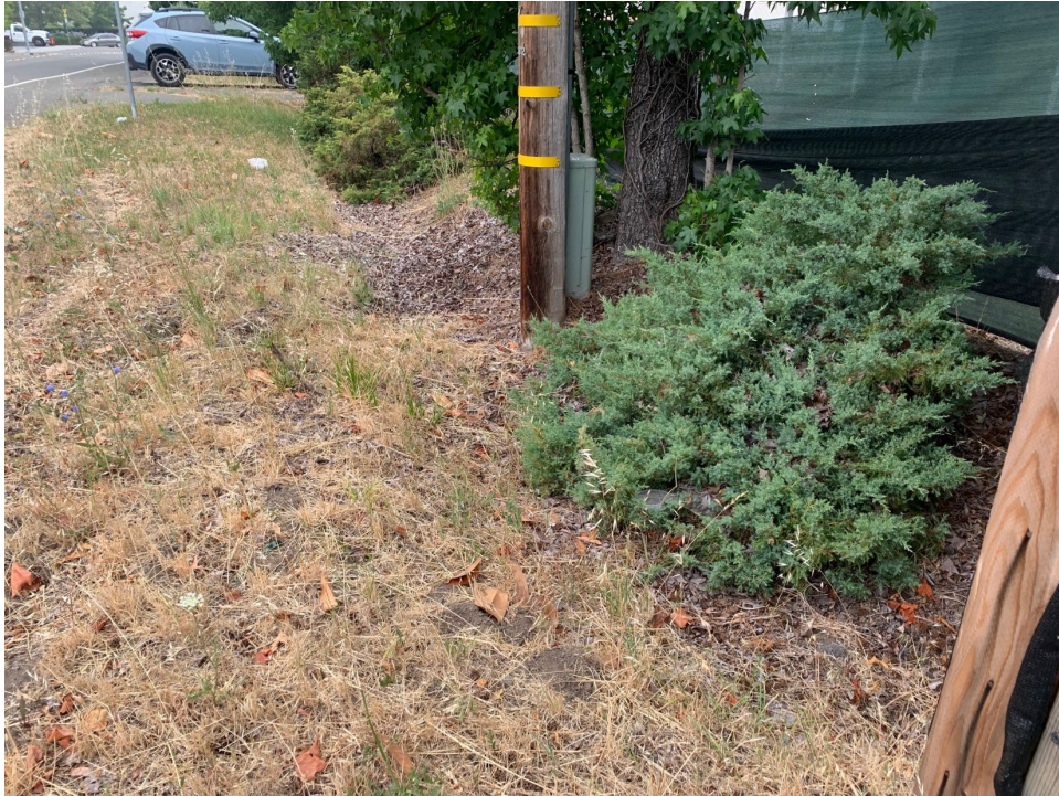
Drainage ditch along Fresno Avenue.
