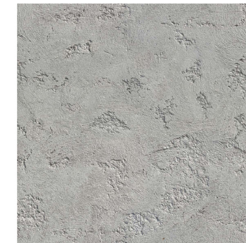
TEXTURED STUCCO EXTERIOR WALL BASE, AND EXTERIOR GYM WALLS
