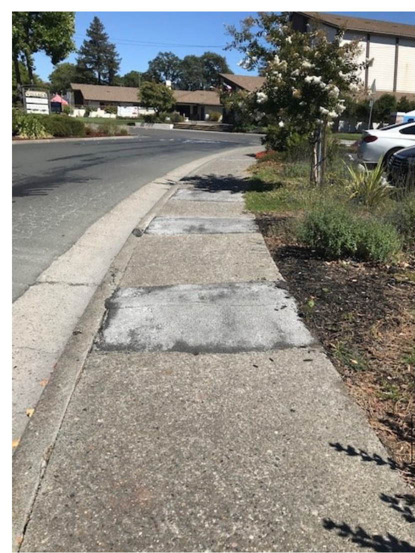
4. SIDEWALK ON PATIO DRIVE - LOOKING WEST REPLACE PATCHED SIDEWALK SECTIONS ON PATIO DRIVE WITH NEW CONCRETE PAVING, AS REQUESTED BY CITY OF SANTA ROSA ENGINEERING, TO MATCH EXISTING WIDTH AND TO RESOLVE TRIP HAZARD FOR PUBLIC
