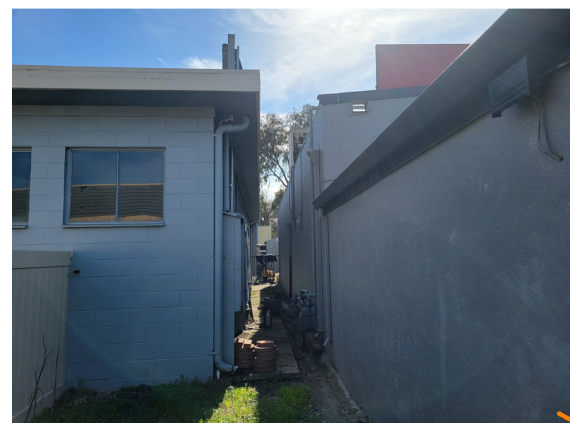
EXISTING CONDITION BETWEEN BOY'S AND GIRL'S CLUB AND RESTAURANT
