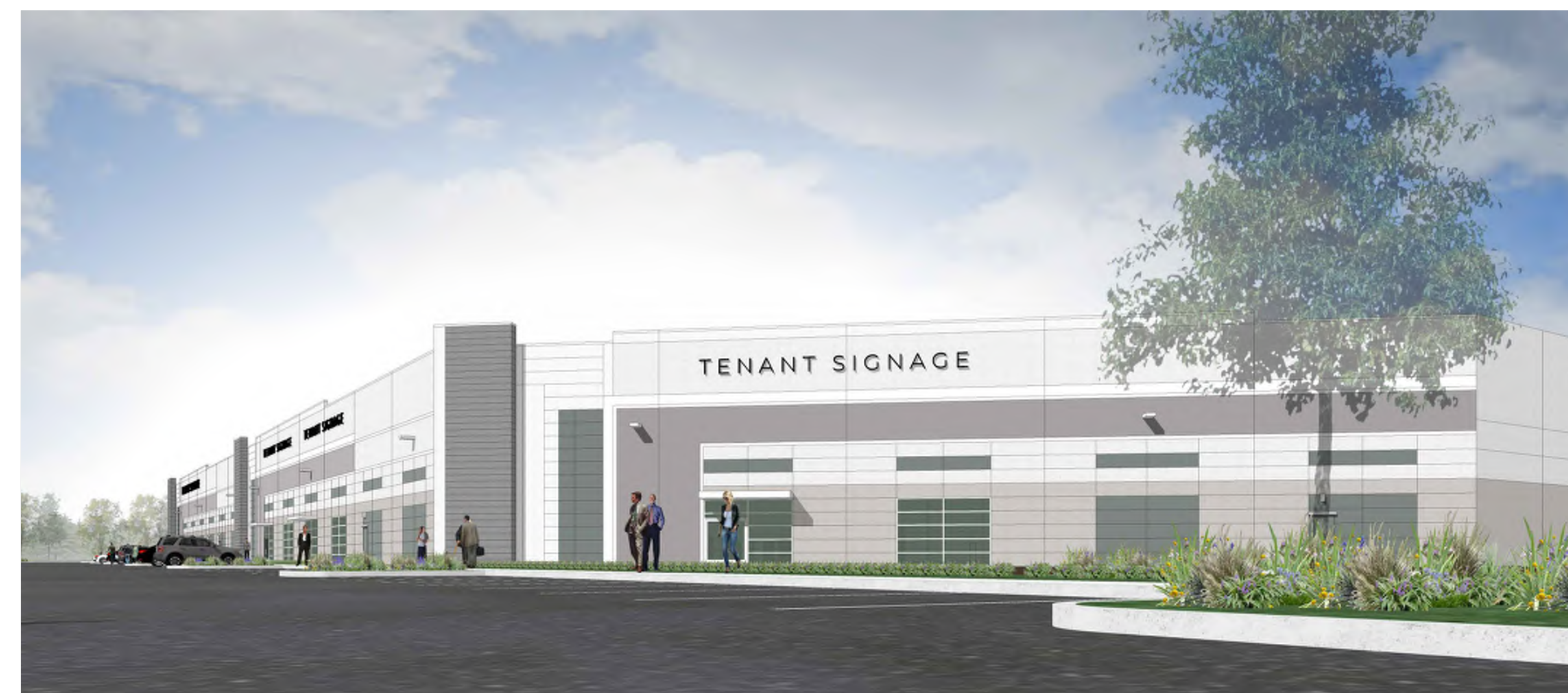
B: VIEW OF NORTH WEST CORNER
